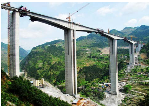
Fig. 1 : Non-prismatic Continuous Beam (Tongzihe Bridge in China)
